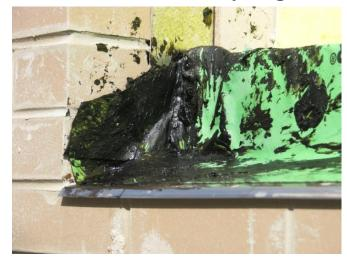
End Dams should be placed UNDER the main flashing run
